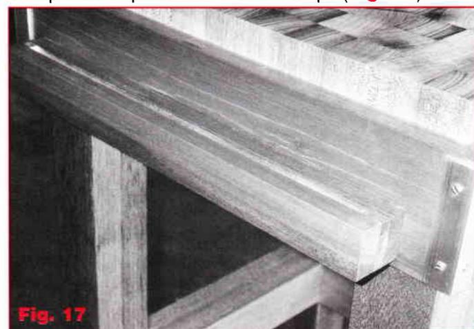
Mount the knife rack with three 8G x 30 mm screws driven from behind one of the sides, which will also conceal the screw heads.
