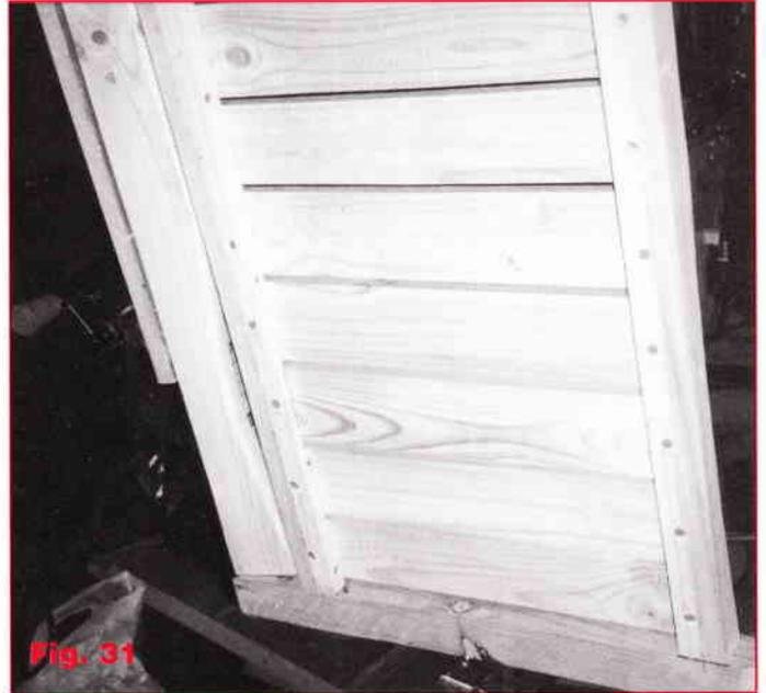
**24** Cut, glue and screw the seat slats (**O**) in place in the same way using 50 mm screws driven from underneath.
